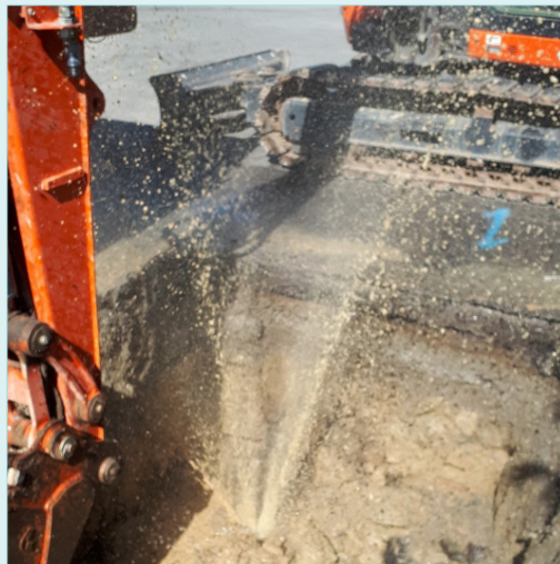
The actual leak photographed during repair
